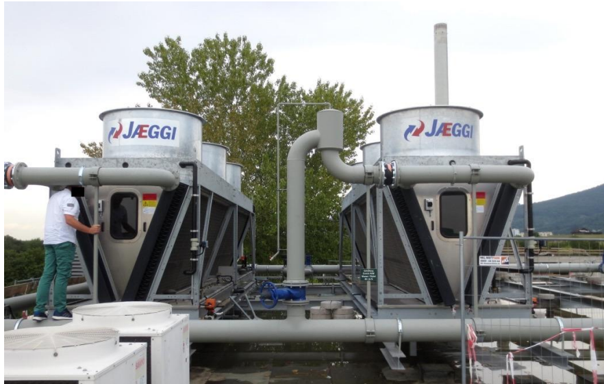
Heat exchanger and wetting on roof of URZ
